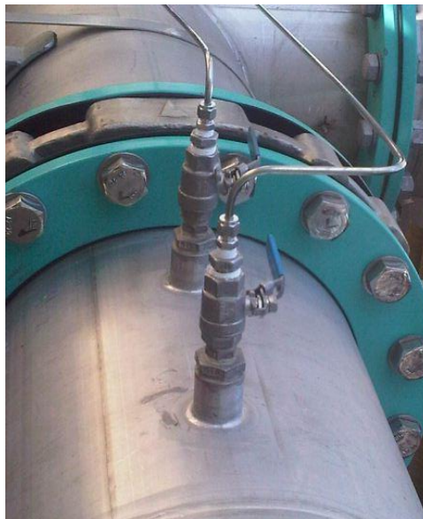
Figure 5 - Ball valve assembly
